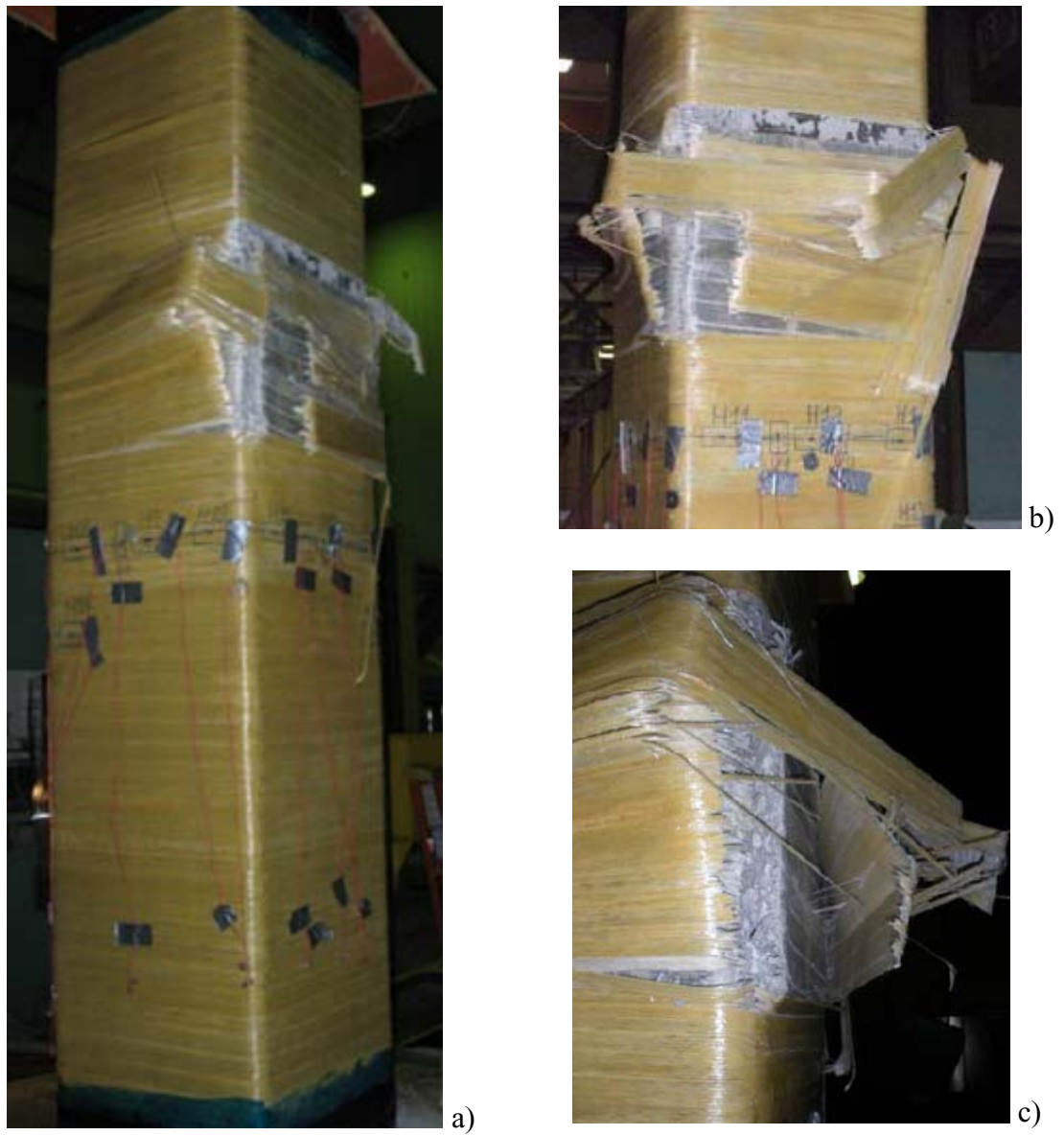
Fig. A - 23: Failure of Specimen S-1-5GA (a-c).
