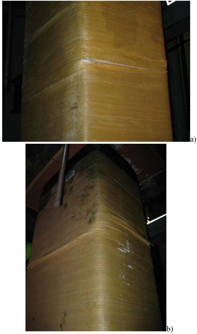
Fig. A - 41: Photographs of failed Specimen HR-8GA (a and b).
